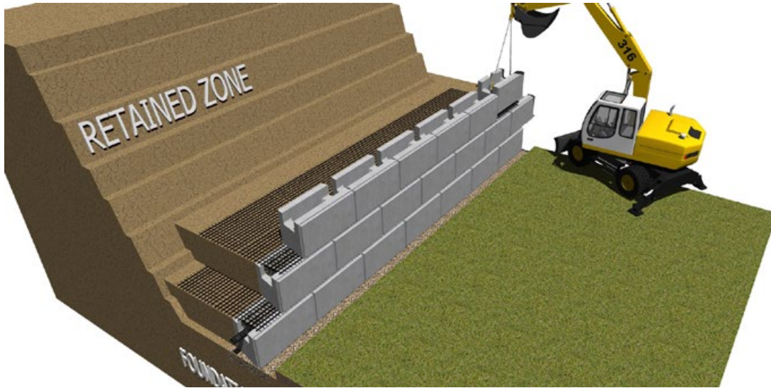
Installing 3rd Row of MaxumStone® retaining Wall Blocks
